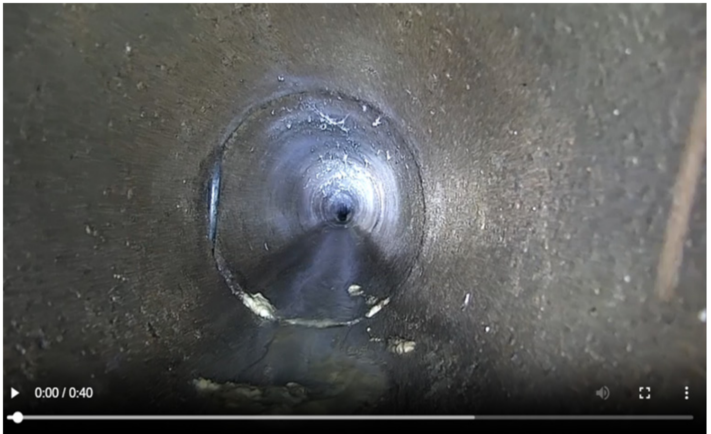
Sewer screening video view into the sewer
