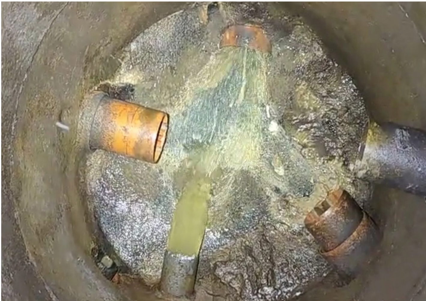
Sewer manhole inspection video
