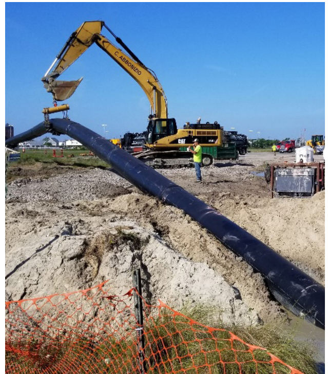
Model Specification MAB-11-2024 provides guidance and instruction for water pressure mini- and maxi HDD installations using HDPE PE4710 pipe.
