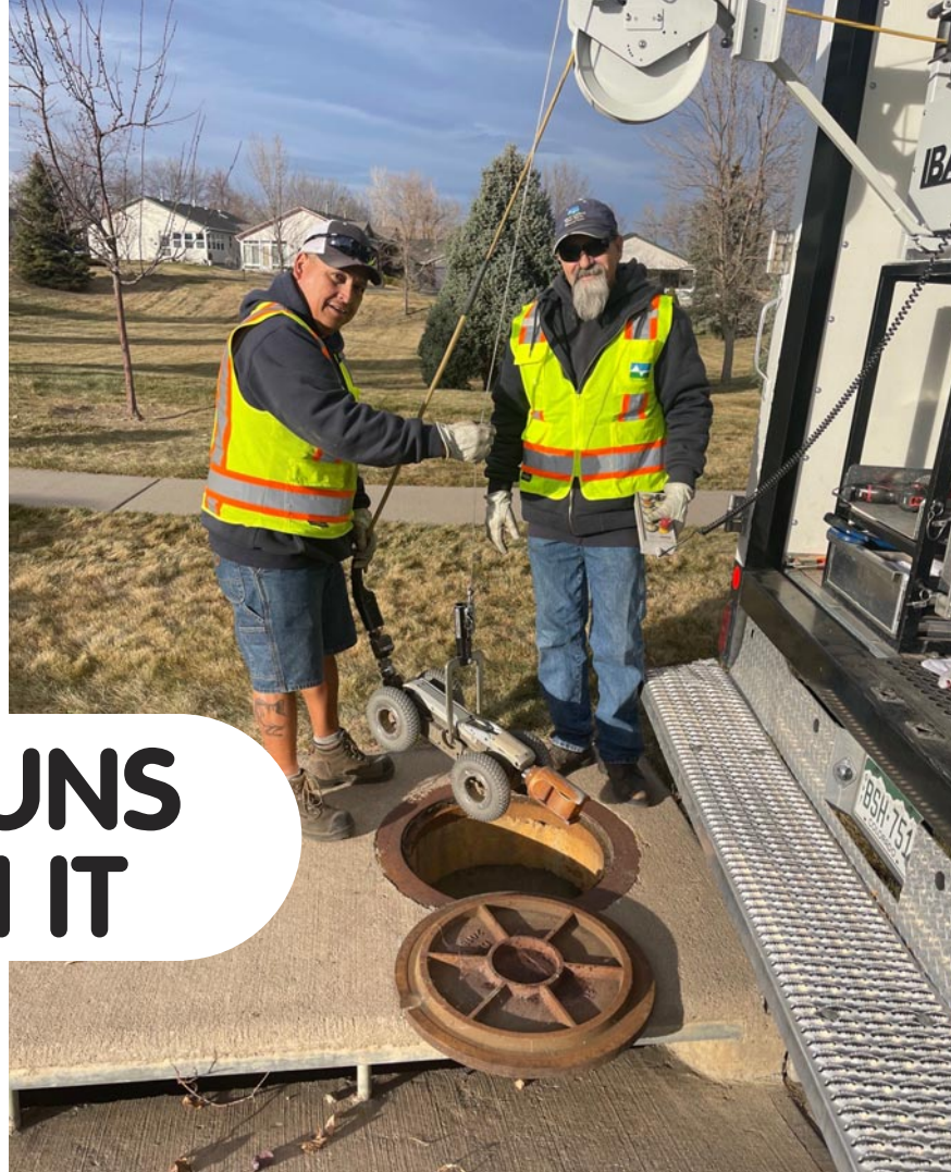
CCTV pipe inspection system gathered more data than anticipated.
