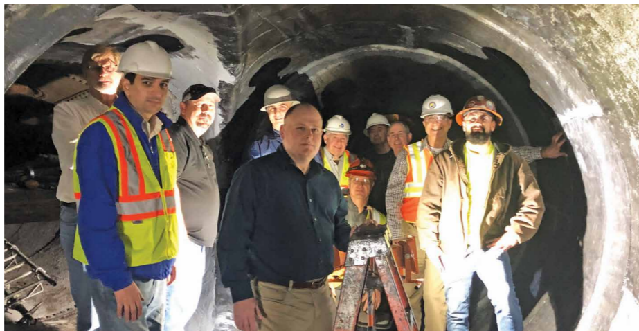
At the top of Lake Lure's dam.
